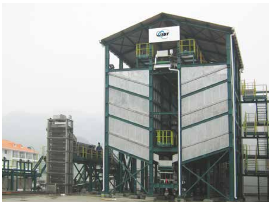
Dry Storage Silos
